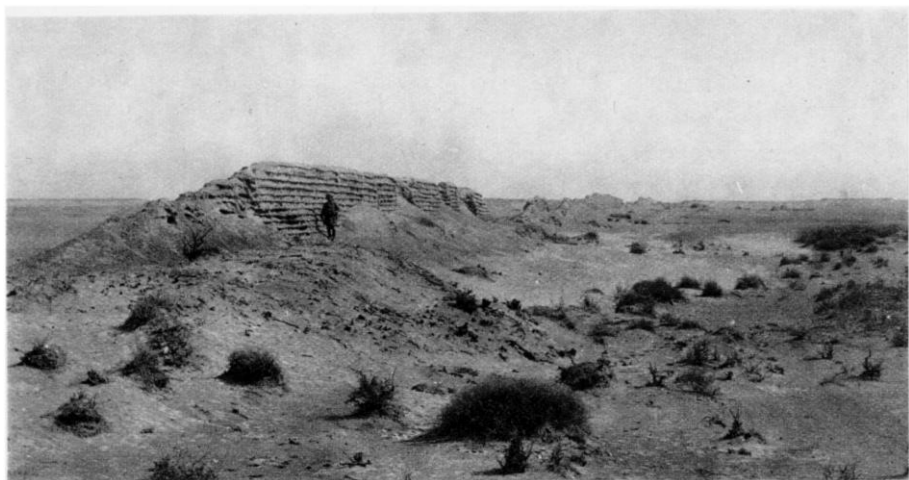
29 ANCIENT CHINESE BORDER WALL BUILT WITH LAYERS OF REED FASCINES, EAST OF WATCH-STATION T.XIII., ON LIMES OF TUNHWANG
